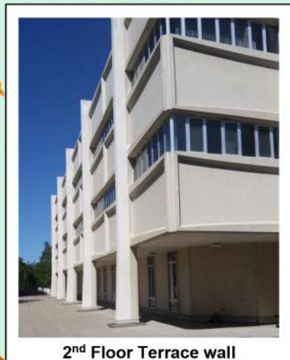
2 nd Floor Terrace wall
