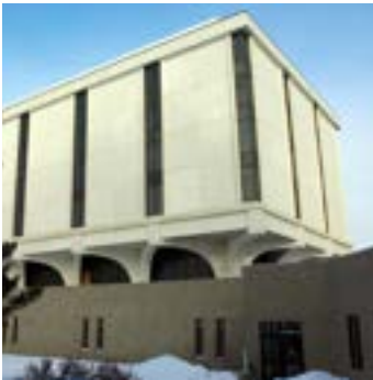
Figure C-51. The Library building has strong design lines that should be respected
