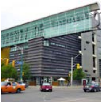
Figure C-14. Gateway buildings establish a sense of place and act as wayfinding features
