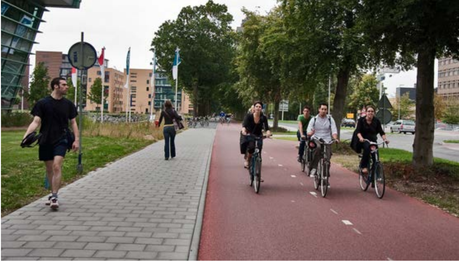
Figure C-62. Off-road dedicated bicycle lanes and pedestrian path
