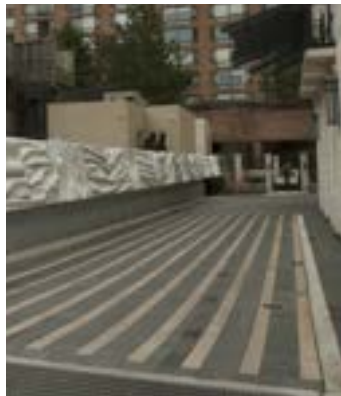
Figure C-16. Service areas should be designed with high quality materials and integrated into the overall public realm
