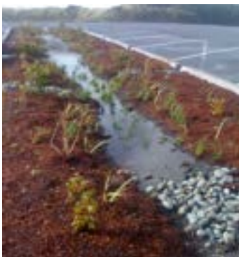
Figure C-21. Bioswales minimize surface runoff
