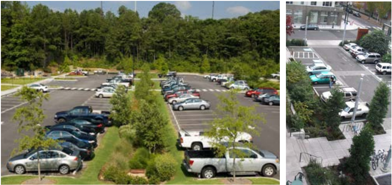
Figure C-17. Bioswales in the design of surface parking lots are multifunctional - they add aesthetic appeal, and mitigate surface water runoff. Bioswales in parking lots can be designed to suit the context, whether more rural (image on the left) or more urban (image on the right). Circulation across the swales can be minimal or numerous depending on the level of activity and do not pose a safety hazard because the swales are very shallow.
