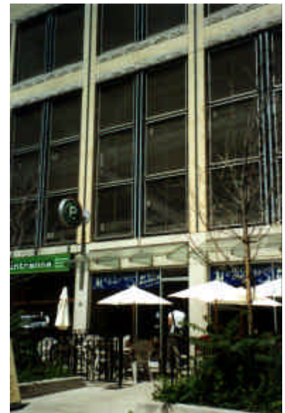
59. A Parking Structure with an Attractive Facade and Ground Floor Retail
