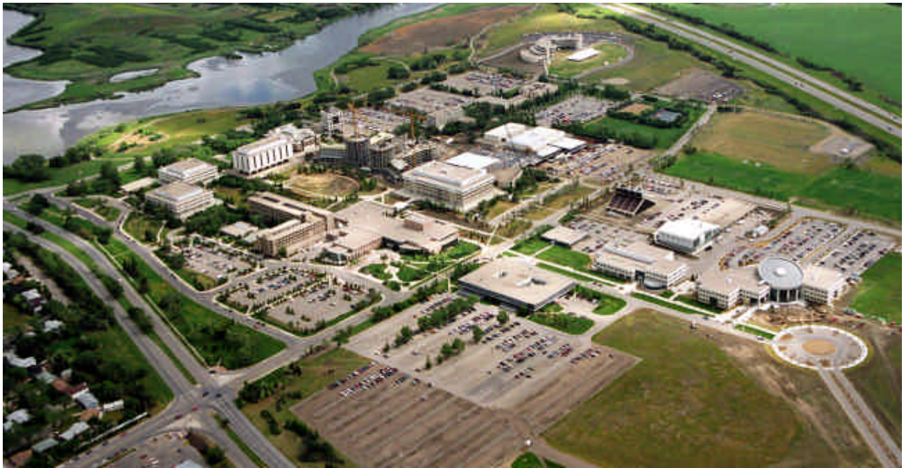
36. Main Campus and Research Park Lands Looking North East - 2003
